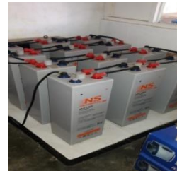
Gambar 32 Batteries OPzS 800
